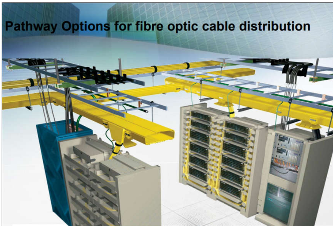
Figure 2 Pathway option Fiber Optic Cable Distribution
